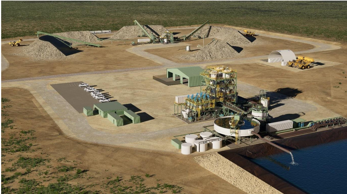
Figure 28: An aerial view render of the proposed Arrowsmith North processing plant and facilities
